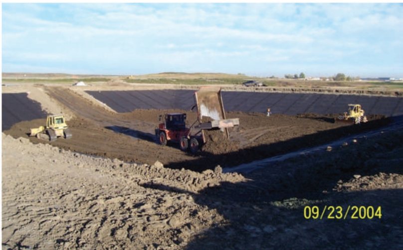
Figure 18.6. Calgary Biocell composite liner construction
