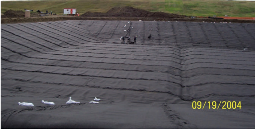
Figure 18.5. Calgary Biocell HDPE liner construction
