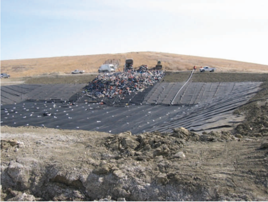
Figure 18.13. Filling operation of Calgary Biocell
