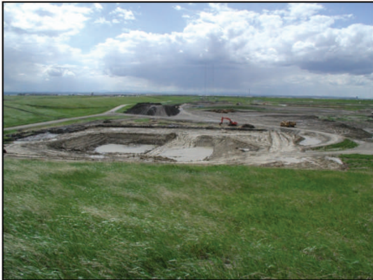
Figure 18.4. Excavation of Calgary Biocell
